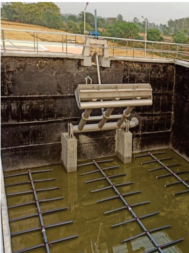
2.5 MLD STP Barwa, PHED Haryana (SBR Decanter and Step Screen)
