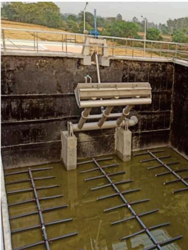
2.5 MLD STP Barwa, PHED Haryana (SBR Deacnter and Step Screen)
